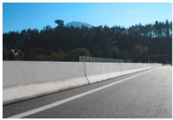
Containment level Working width Impact severity level T3 (covers T2 and T1)
