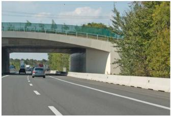
Containment level Working width Impact severity level H2 (covers H1, N1, T3, T2 and T1) W3 (covers W4, W5, W6, W7 and W8) ASI B
