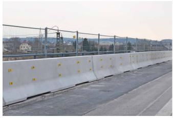
Containment level Working width Impact severity level H2 (covers H1, N1, T3, T2 and T1)
